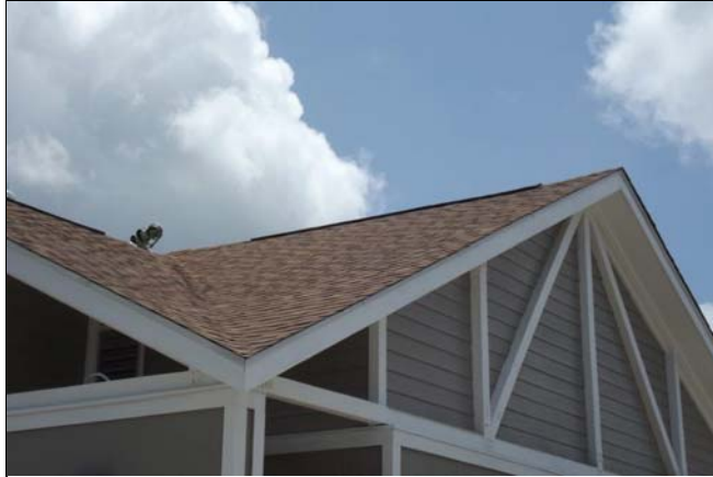
7. Roofing systems consist of asphalt shingles of various ages.
