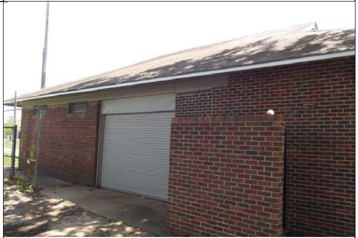
4. The Herndon Park Maintenance is clad with brick.
