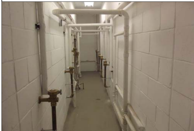
9. The utility chase area of the new toilet room building.
