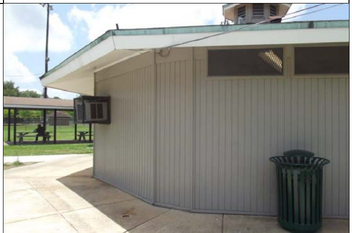
6. The concession stand is clad with wood panel siding.
