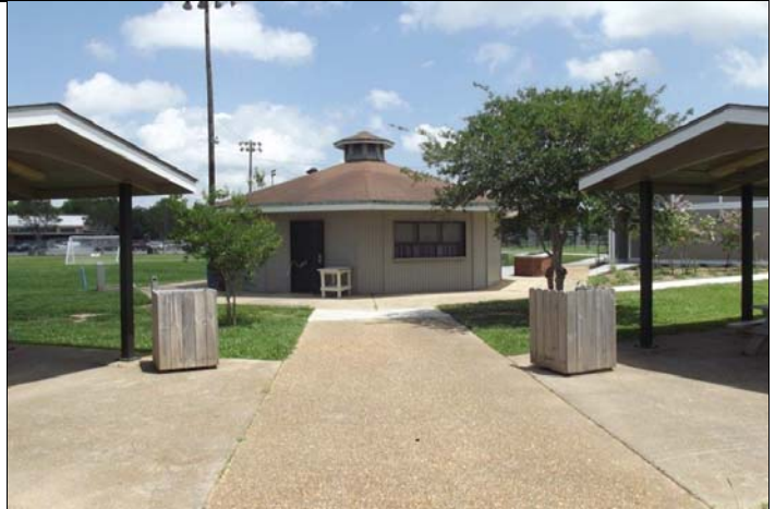
2. The Subject also includes the concession stand building.
