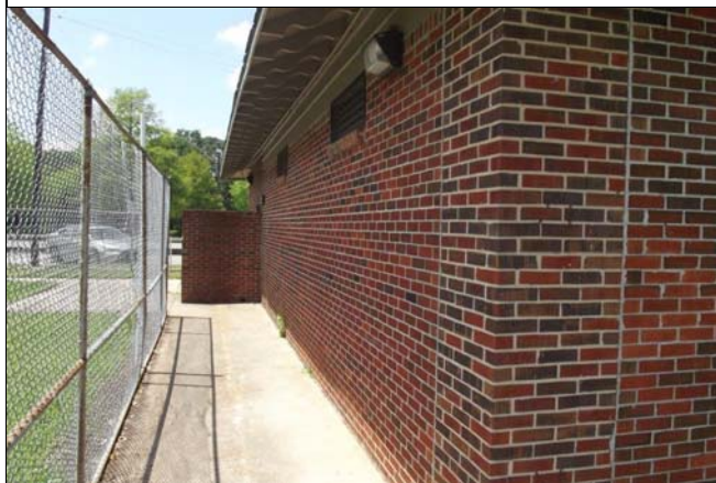
5. Concrete sidewalks are located alongside the building.
