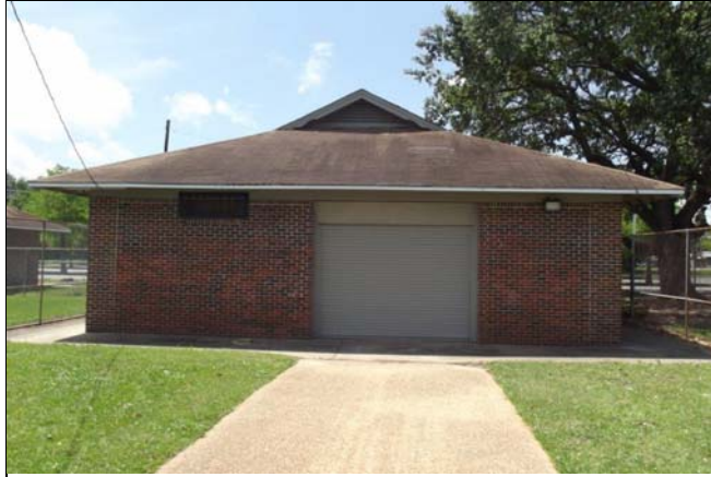
1. The Herndon Park maintenance office as viewed from the rear.
