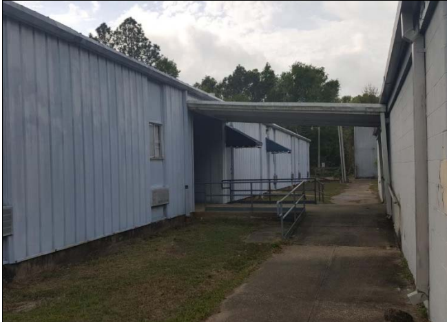
7. Classroom 2 is a pre-manufactured metal building connected by a steel canopy.
