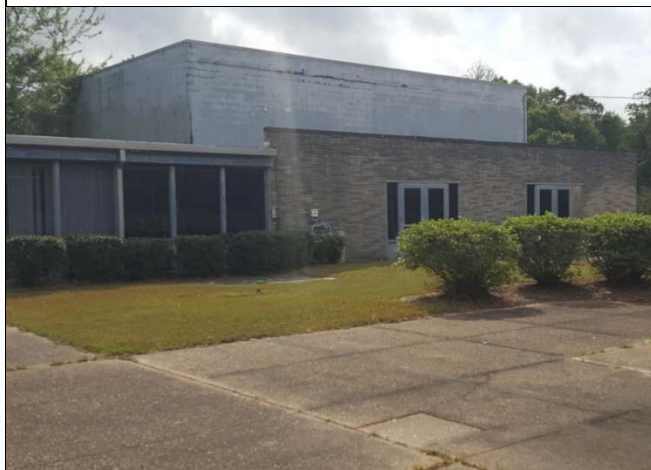
5. The main building is CMU faced with stone on the front elevation.
