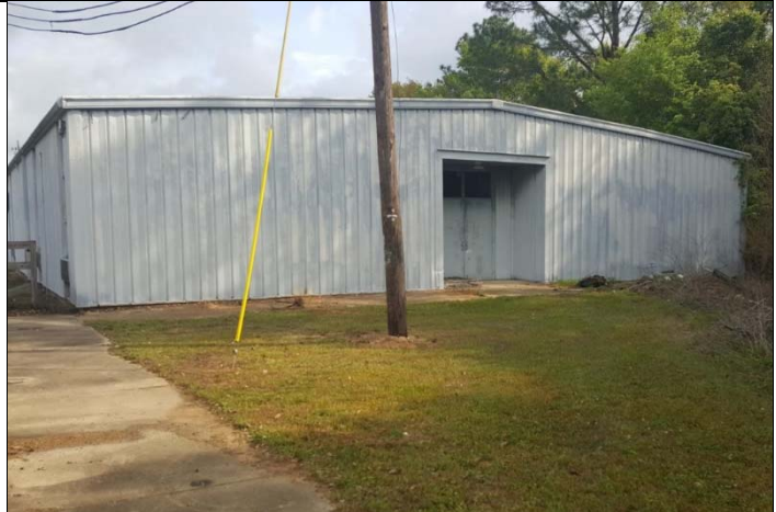
8. Classroom 2 primarily has painted metal panels for the walls and roof.
