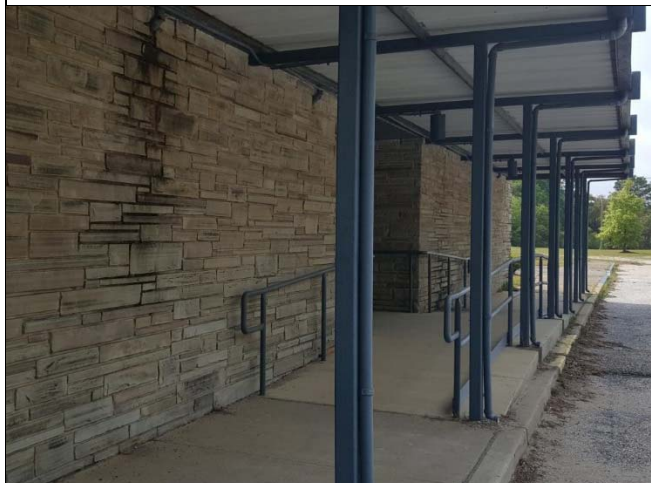
3. There are concrete sidewalks and ramped walkway at the front entrance.
