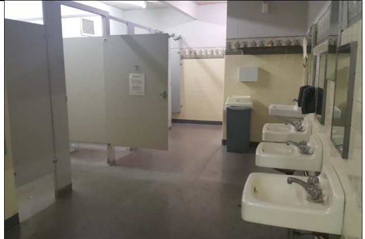
14. Two large multi-user toilets are located in the Classroom 1 building.
