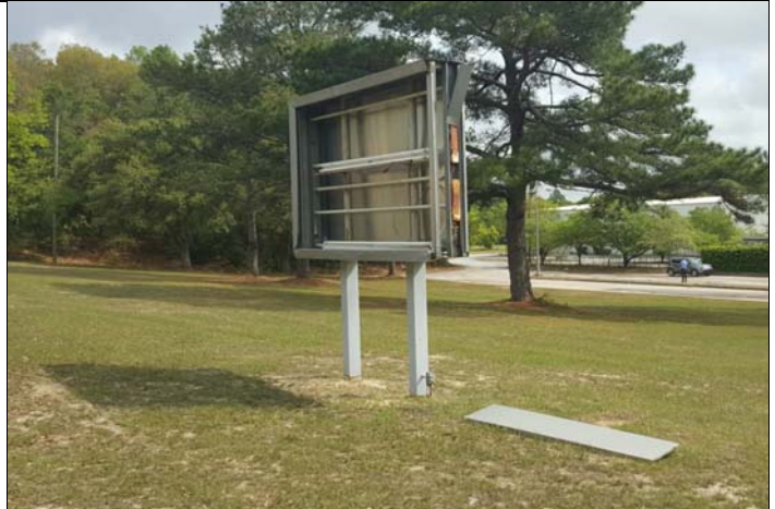
2. The damaged sign located along the front edge of the property.
