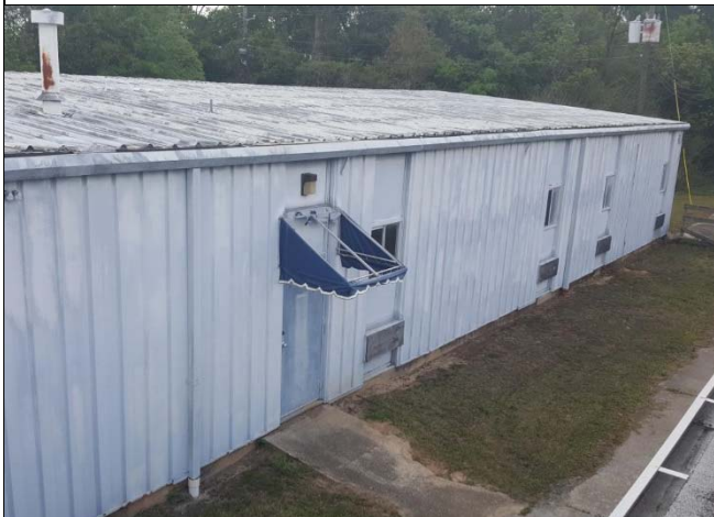
11. Classroom 2 has a low slope metal roof drained by gutters and downspouts.
