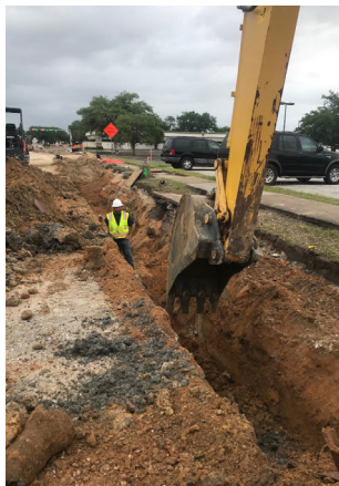
Crews dig a trench for a 16-inch water main.
