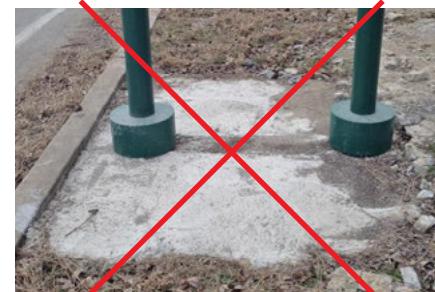
NOT Acceptable Footer Detail
