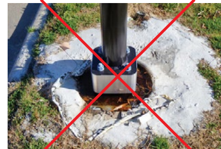
NOT Acceptable Footer Detail
