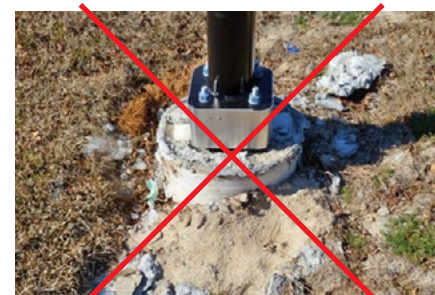
NOT Acceptable Footer Detail
