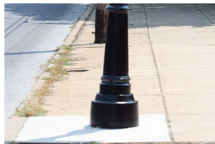
Acceptable Footer Detail
