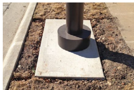
Acceptable Footer Detail
