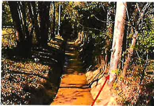
Buffer Area Encroachments
