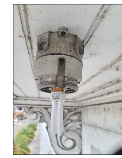
2 TYPICAL EXTERIOR LIGHTING FIXTURE TO BE REMOVED AND REPLACED NEW NOT TO SCALE
