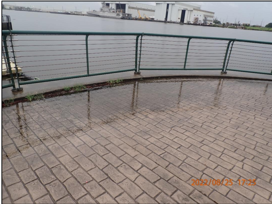
Photo 4 Areas of settlement adjacent to south sheet pile bulkhead. On structure, looking northeast.
