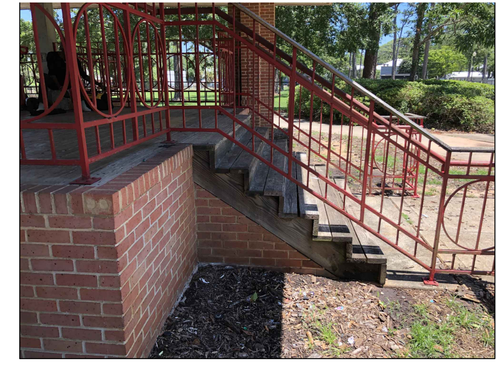
PAVILION PHOTO 04 • REMOVE EXISTING STEPS. PREPARE FOR NEW CONCRETE SLAB.
