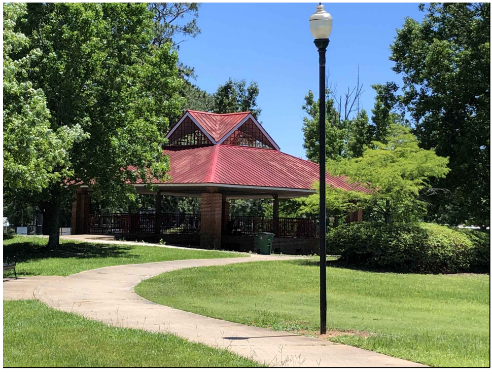
PAVILION PHOTO 01 • OVERALL VIEW OF PAVILION
