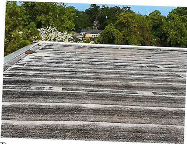
The gymnasium roof, looking across the southwest corner.
