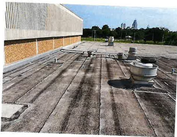
Looking northward across roofs 2 & 3, with the gymnasium wall to the left.
