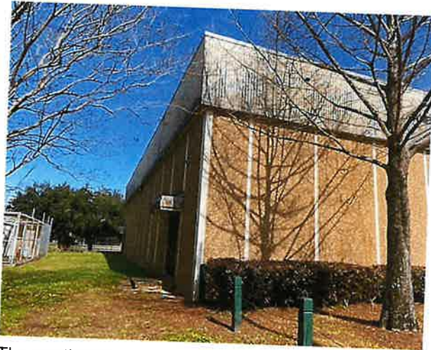
The southwest corner of the building.
