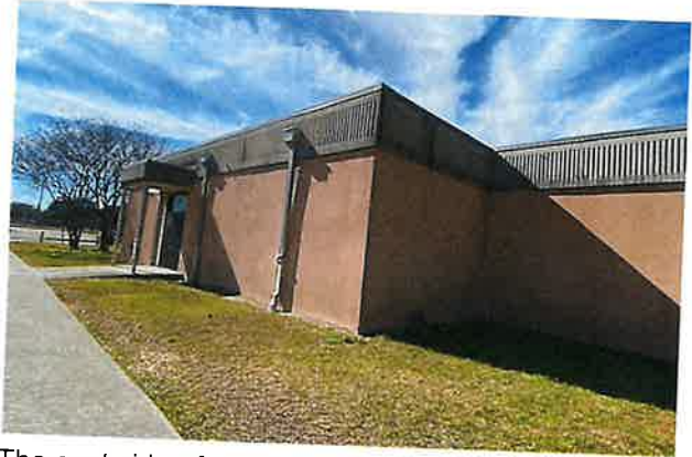
The east side of the building, with the canopy over the east entry.
