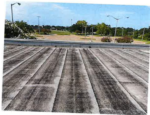
Standing on Roof 2, looking southward.
