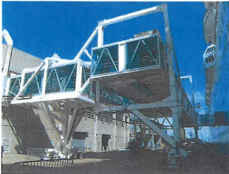
Seaport Passenger Boarding Bridge HYDRA MS1 at Alabama Cruise Terminal
