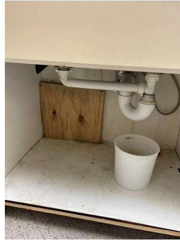
2. Underneath Leaking Kitchen Sink with Evidence of SVMG. Behind Wood Board is SVMG in Void Space
