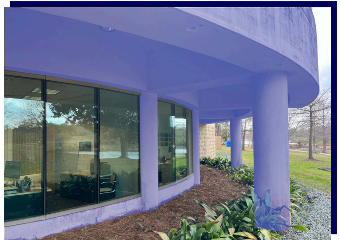
Office facade below entrance
