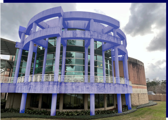
Front facade/entrance to Museum
