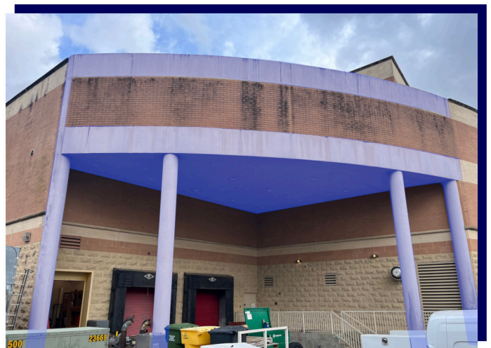
Rear loading dock
