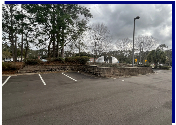
Illustration of retaining walls to be cleaned
