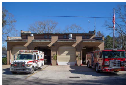
MELTON STATION, #8 Engine 8, Rescue 8, District 1, Technical Rescue 8, Water Rescue 8
