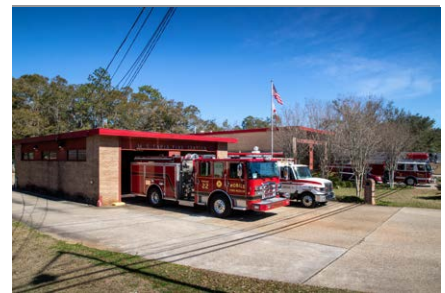
TAPIA STATION, #22 Engine 22, Rescue 22, Truck 5
