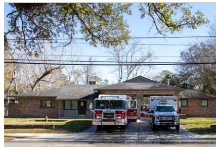
TOULMINVILLE STATION, #14 Engine 14, Rescue 14
