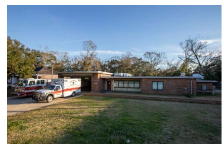
SIRMON STATION, #23 Engine 23, Rescue 23
