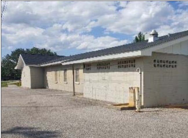
3. The west elevation is homogenous with the other sides of the building.
