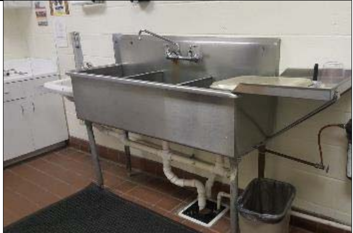
8. A small warming kitchen is located at the rear of the building.
