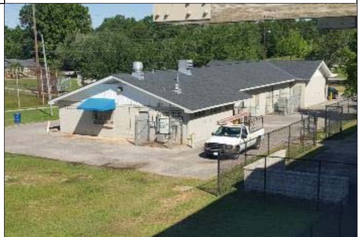
6. The roof is asphalt shingles reportedly about 1 year old.
