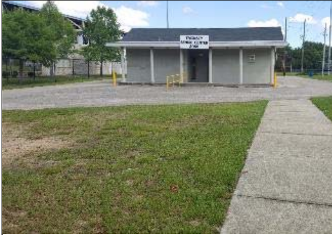
1. The building is a single story structure accessed by an asphalt drive and concrete sidewalks. A ramp system with metal railings is provided at the front entrance.
