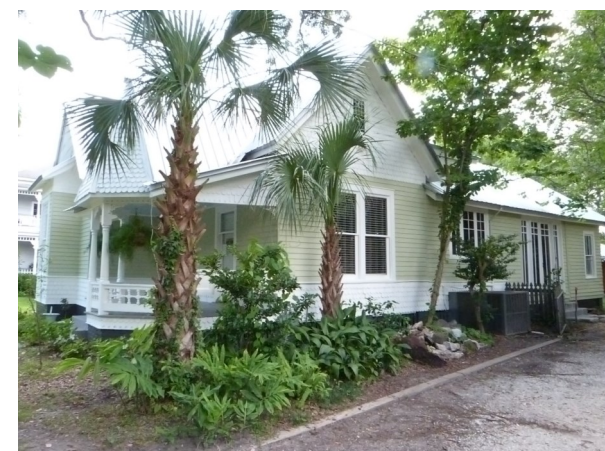
113 S. Georgia Avenue Gray and Julia Fobes Lossing-Fobes, 1896
