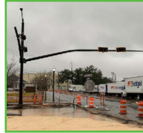
Crews have installed the mast arms for traffic lights.
