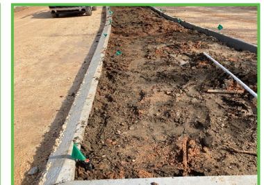
Irrigation and topsoil have been placed in the medians.
