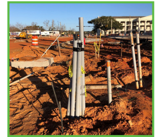
Conduit stubbed up at Springhill Ave.
