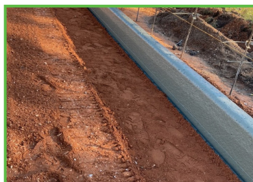
Crews continue to work on curbs around the roundabout.
