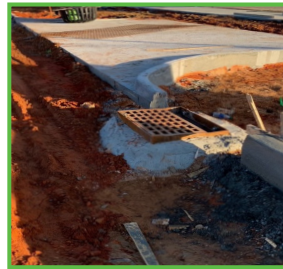
Storm sewer systems are being installed with a crushed aggregate base.
