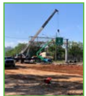
Crews removing the sign bridge.
