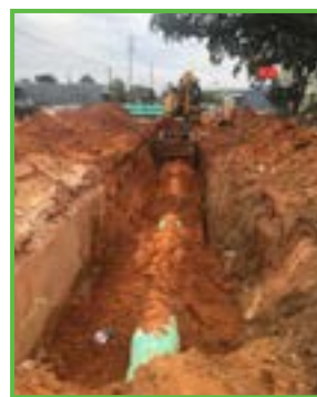
New water line in place and trench being backfilled.
