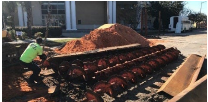
● Staging the augers for boring
