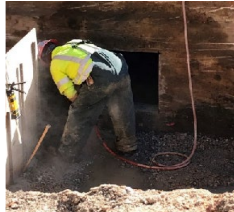
● Working in a box culvert
