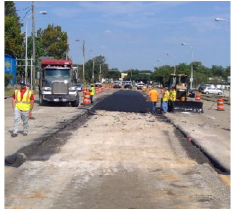
● Laying the cross over
