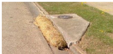
Protecting the stormwater inlets on Broad St.
