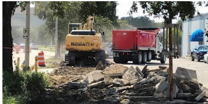
● Hauling off concrete after demolition
