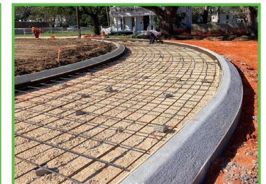
The center of the roundabout is almost ready for landscaping.
