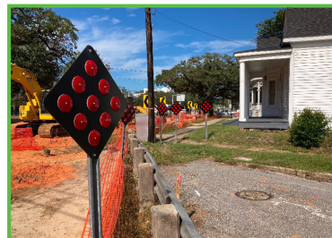
Reflective road signs have been installed to increase safety around the work zone.
