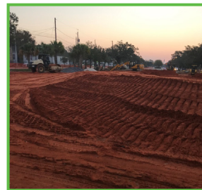
Material is brought in to build up the Broad and Canal Street intersection for the roundabout.
