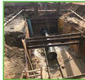
Crews use the jack & bore process to install a 24" waterline at Springhill Avenue.
