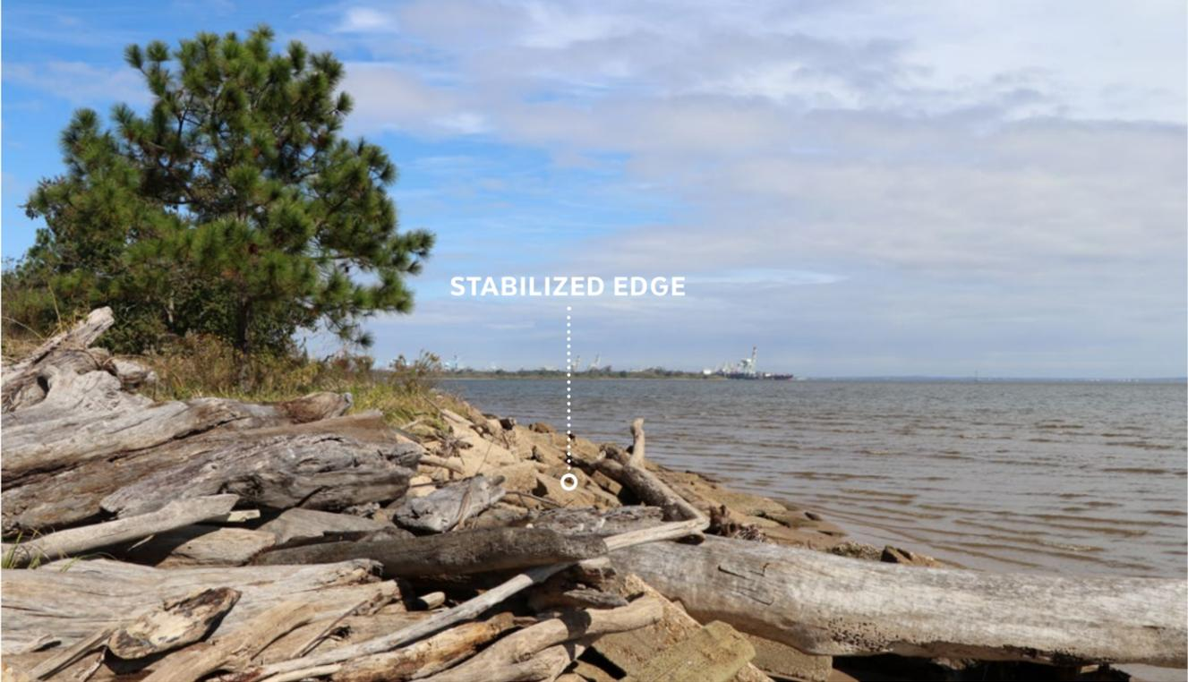
**VIEW 1** The edge is stabilized with concrete rubble and pockets of vegetation. Driftwood accumulates along the edge.
